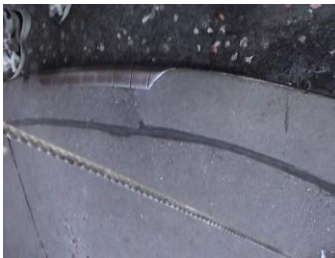
Metal cap stone pavement
