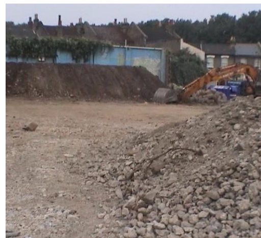
Building site; behind the house where I live.
